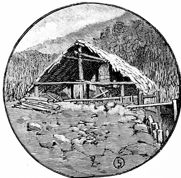
FIG. 2.—NATIVE CHINESE TIN-STAMPING MILL ON THE KUANTAN, MALACCA.
